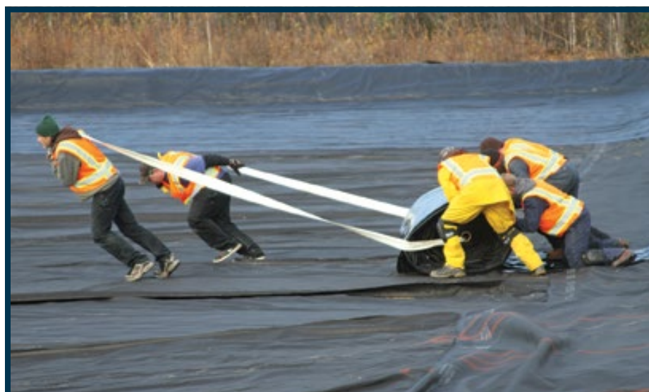
The impermeable liner is spread for construction of the tank.
